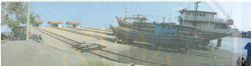
Gambar 2.11 Sloped slipway (Sumber: www.google.com , 2016)
