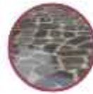
Paving batu alam
