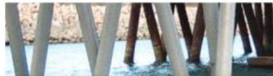
Gambar 2.33: Pondasi Bore Pile
