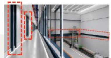
Building Main Structure
