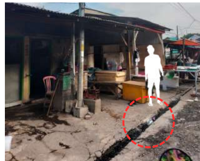
Gambar 6: Drainase pasar ikan
