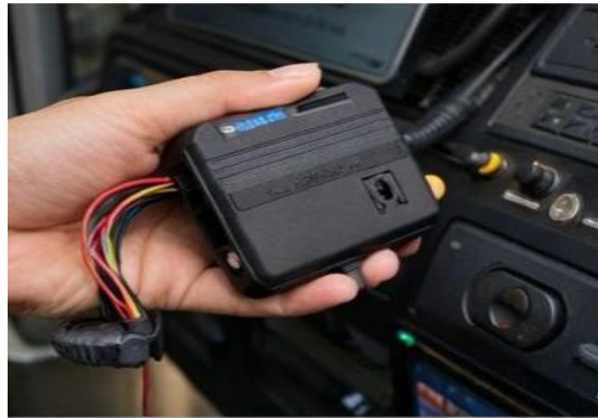
Figure 4.1 Installation of GPS Tracker
