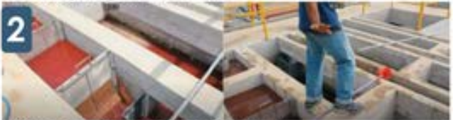
2 Oil Separation + Grid Chamber
