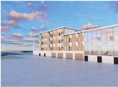
PENGUNAAN KINETIC FACADE DI AREA FIA CONTROL CENTRE
