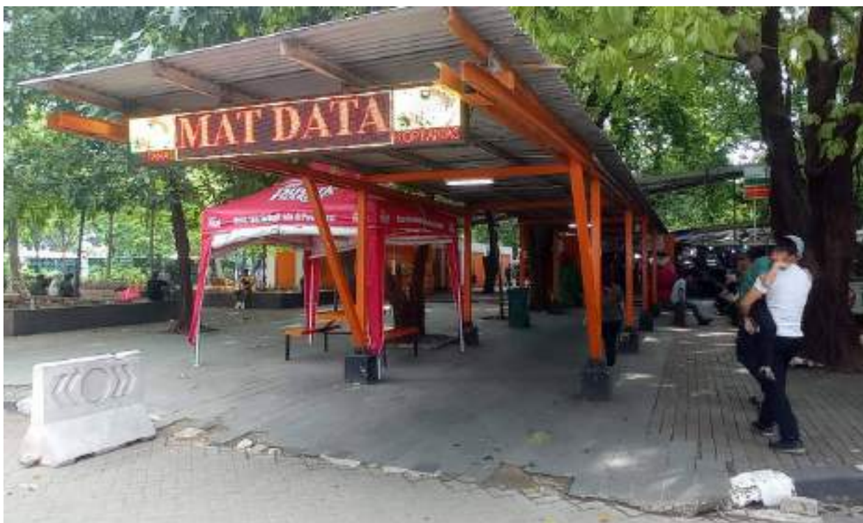
gambar 4.9 interior rest area km456
