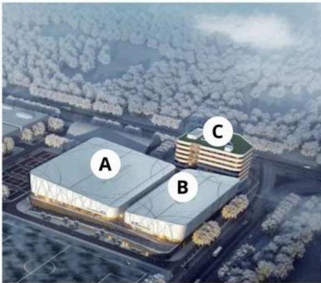
Gambar 16. Tata masa bangunan National paralympic Training Venue
