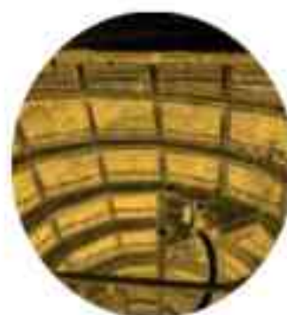
RING BEAM STRUCTURE
