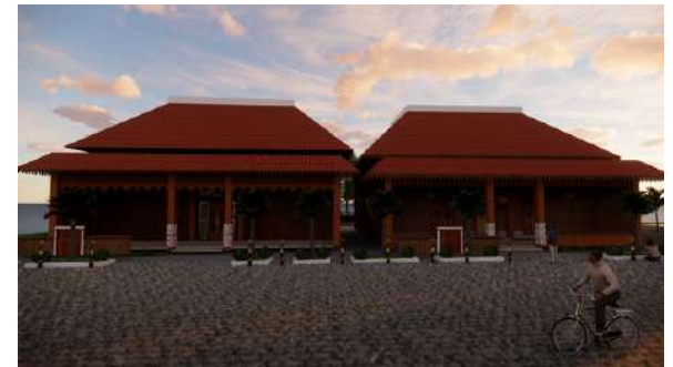
GUEST HOUSE & KAFETERIA
