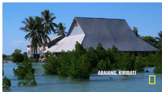
Figure 1.4 A flooded house. (minute 00:40:58)
