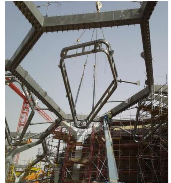
Gambar 2.44 Struktur Utama KAPSARC Sumber: KAPSARC – Tensile Fabric Building Skin,[37]
