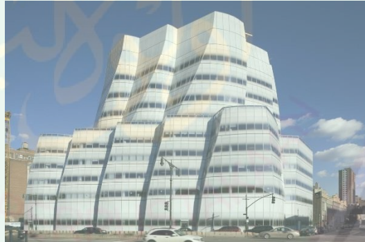
Gambar 2.42 IAC Building Low (sumber: Bintang Panca Aditya, 2010)
