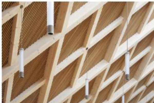
Struktur atap menggunakan Glulam di Ibstock Place School, Roehampton
