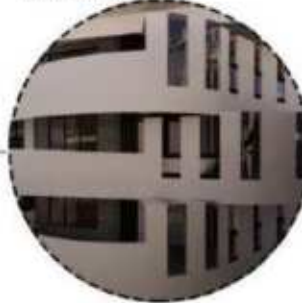
BALCONY DAN SELASAR (IN BUILDING)
