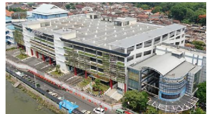
Gambar 2.12 Terminal Intermoda Joyoboyo, Surabaya (Sumber: https://www.mongabay.co.id/2020/03/13/green-terminal-intermoda-pertama-di-indonesia-ada-di-surabaya/ )
