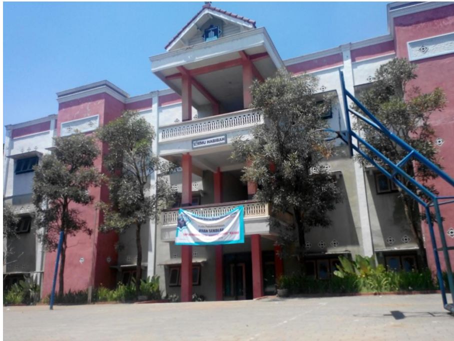
Picture 1. School building of SMP Ar-Rohmah Putri Boarding School
