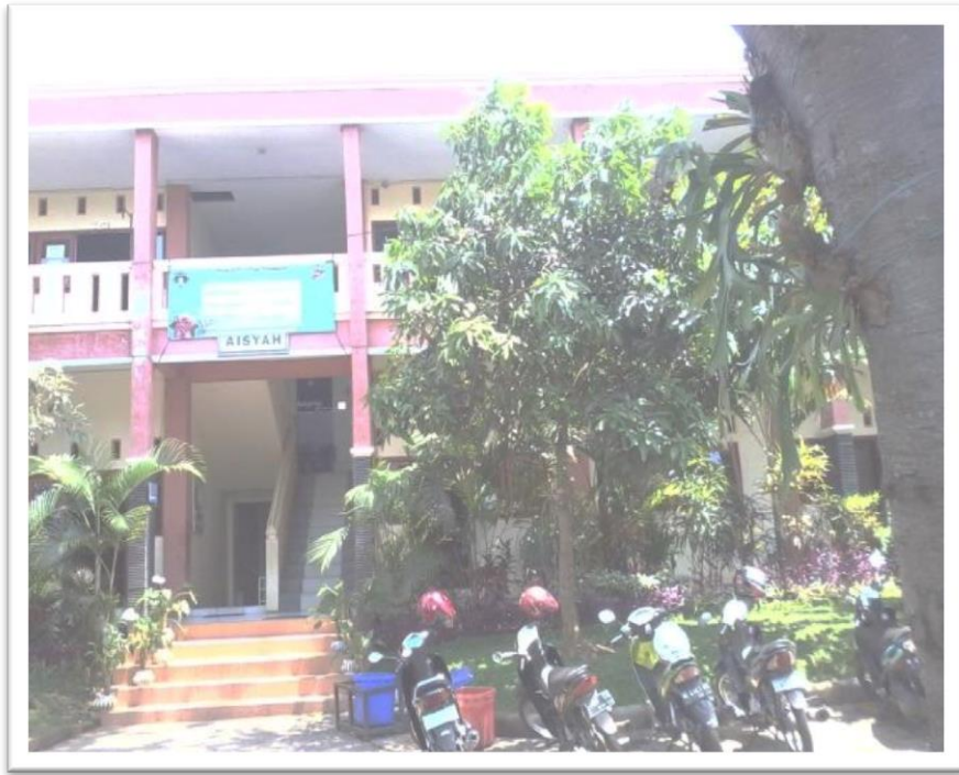
Gambar 7 : Kantor SMP Ar-Rohmah Putri “BOARDING SCHOOL” DAU Malang
