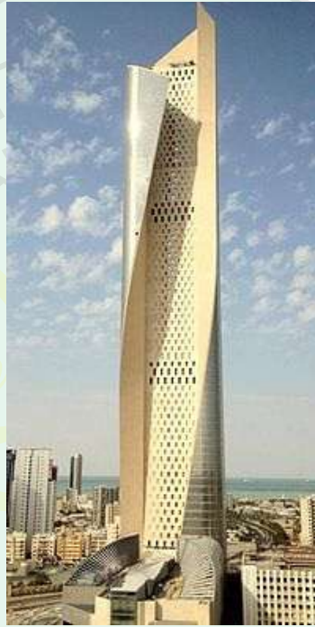
Gambar 2.39 Al Hamra Firdous Menara (Sumber : http://en.wikipedia.org/wiki/Al_Hamra_Tower )
