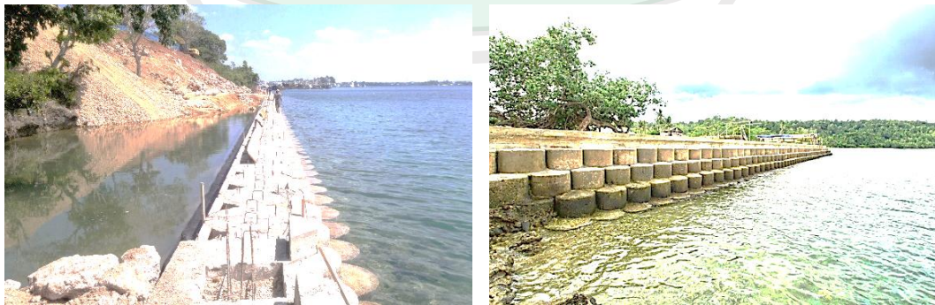
Gambar 6.10. Ilustrasi Retaining wall Sumber: Google 2016
