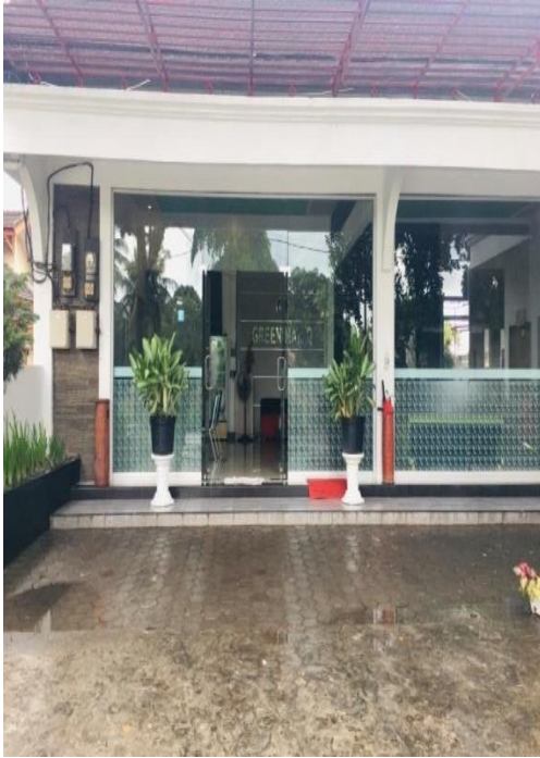
Figure 10 Hotel parking area
