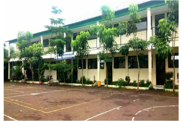
Bangunan SMP Bahrul Maghfiroh
