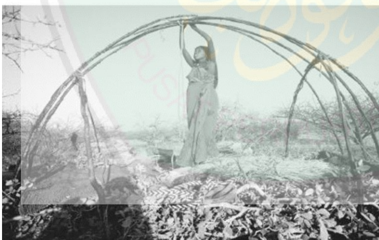
Figure 2.18 Ongoing building of Somali traditional house
