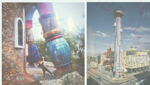
Gambar 2.12 Detail Eksterior Bangunan Maishima Incineration Plant
