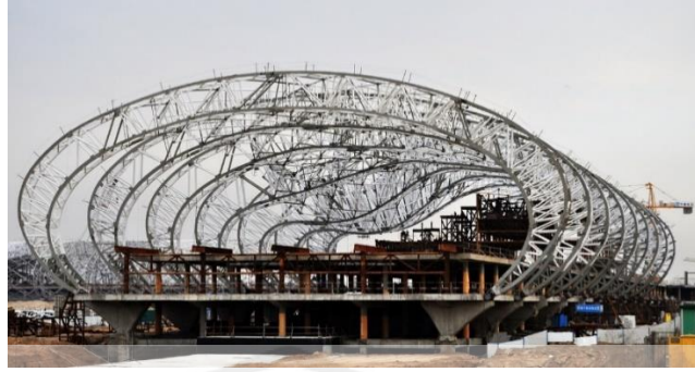
Figure 2.21; Shenzhen Bao'an International airport, China - Focus structure; https://www.arketipomagazine.it/en/shenzhen-baoan-international-airport-china-focus-structure/
