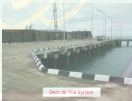
Gambar 2.24 Deck Pile System
