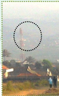
Gambar 4.8 Tower telepon Sumber : Hasil survey (2013)
