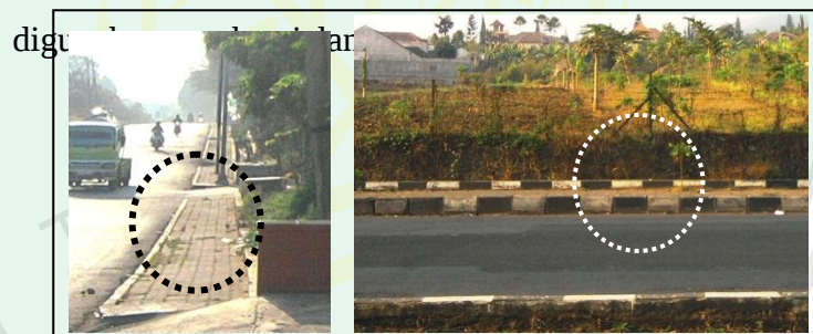
Gambar 4.10 Drainase tertutup Sumber : Hasil survey (2013)
